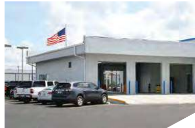
Gutters and Downspouts
