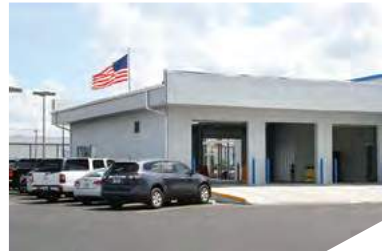
Gutters and Downspouts
